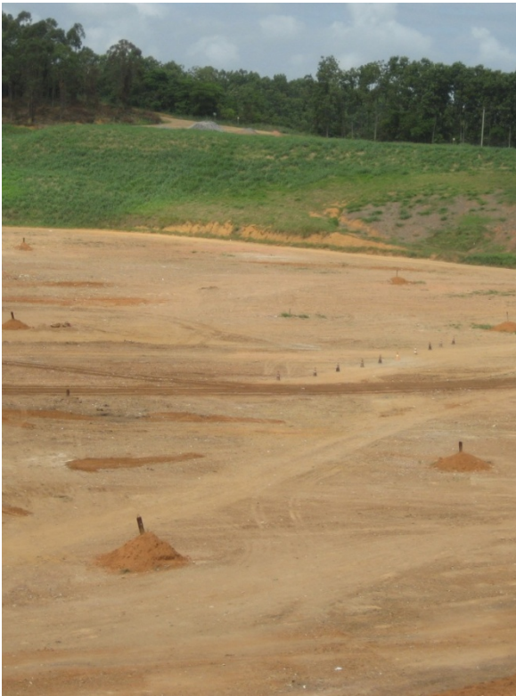
Figure 8. Venting Wells
