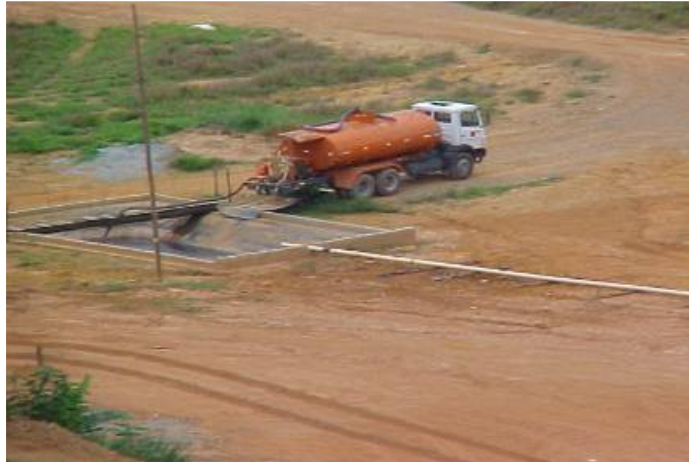
Figure 7. Leachate Collection Pond
