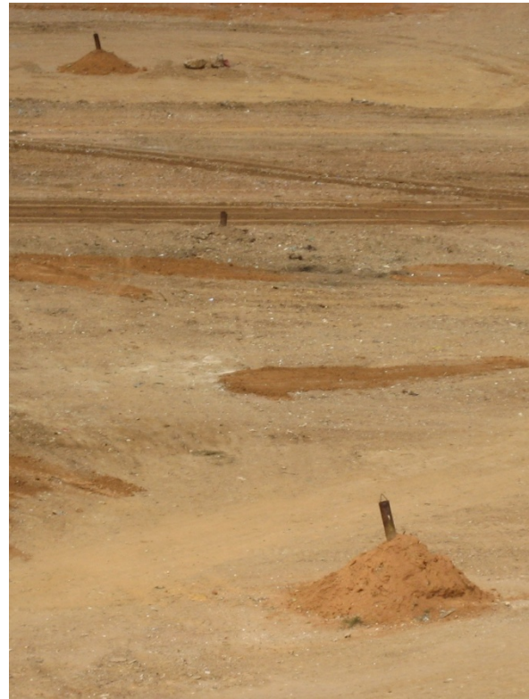
Figure 9. Venting Well
