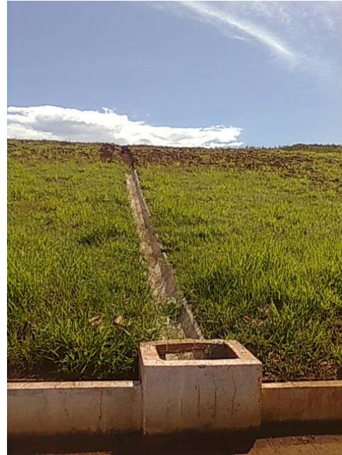
Figure 6. Leachate Drainage Trench
