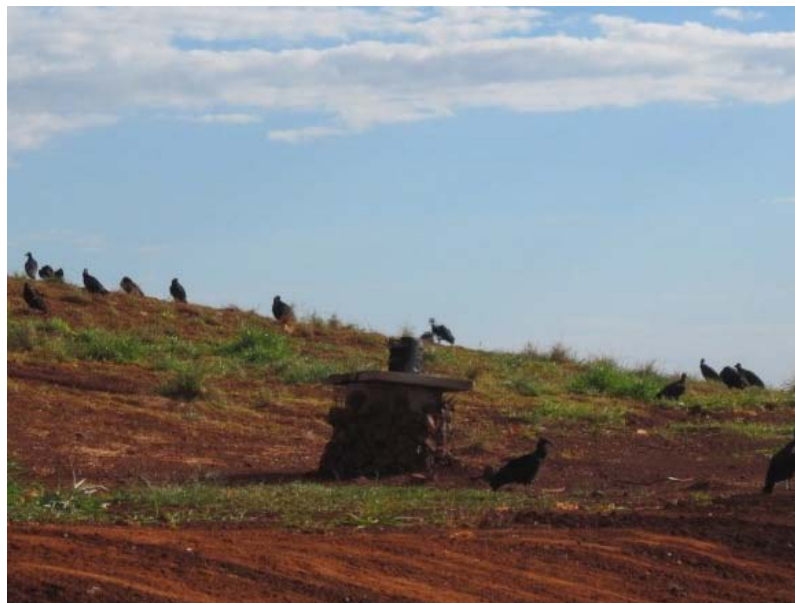
Figure 10. Venting Well with Flaring of LFG
