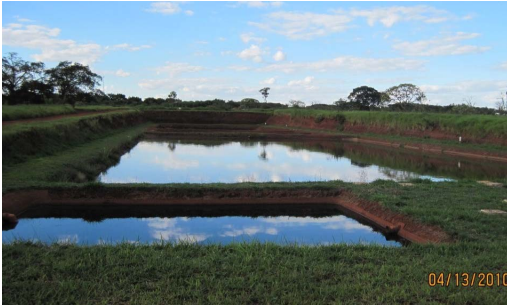
Figure 7. Leachate Evaporation Lagoons
